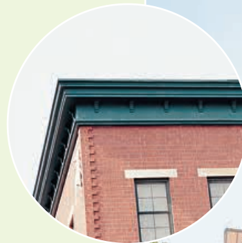
Moulding with brackets, pre-finished in the factory
